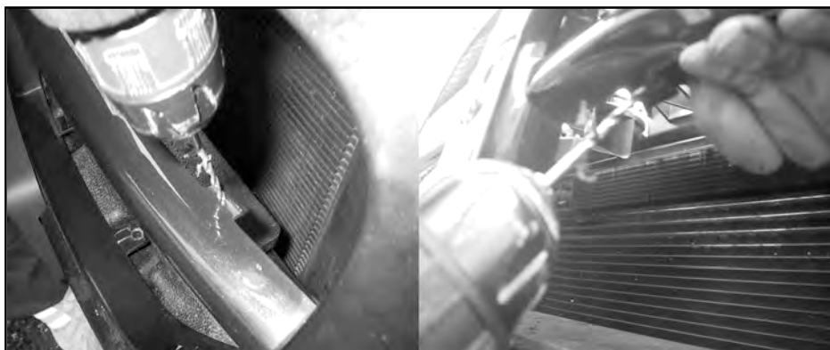
Figure 6. Drill holes on inner-arm clips to use for fastening new grilles.
